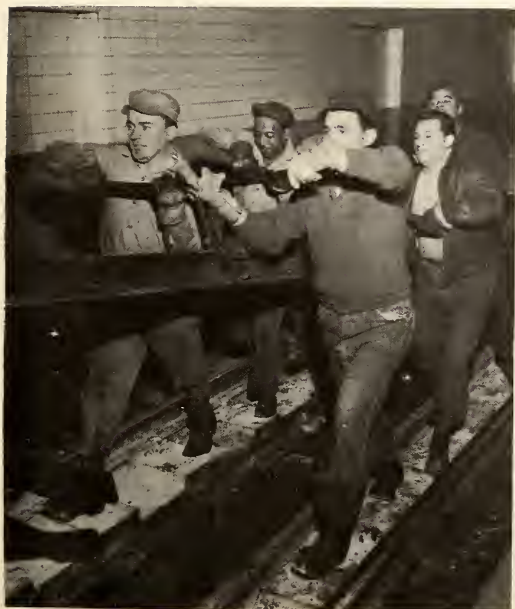
TRACK REPAIR MEN
